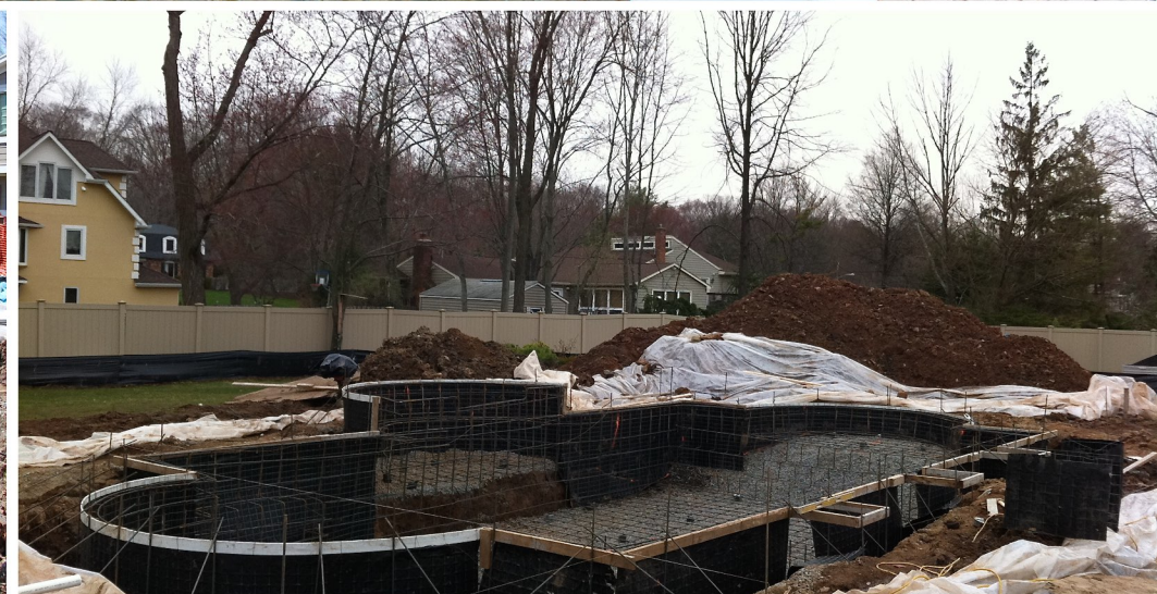
Remove old liner pool and replace with custom-designed 850 square foot gunite masterpiece. From demolition to swimming, this project took approximately ten weeks.
