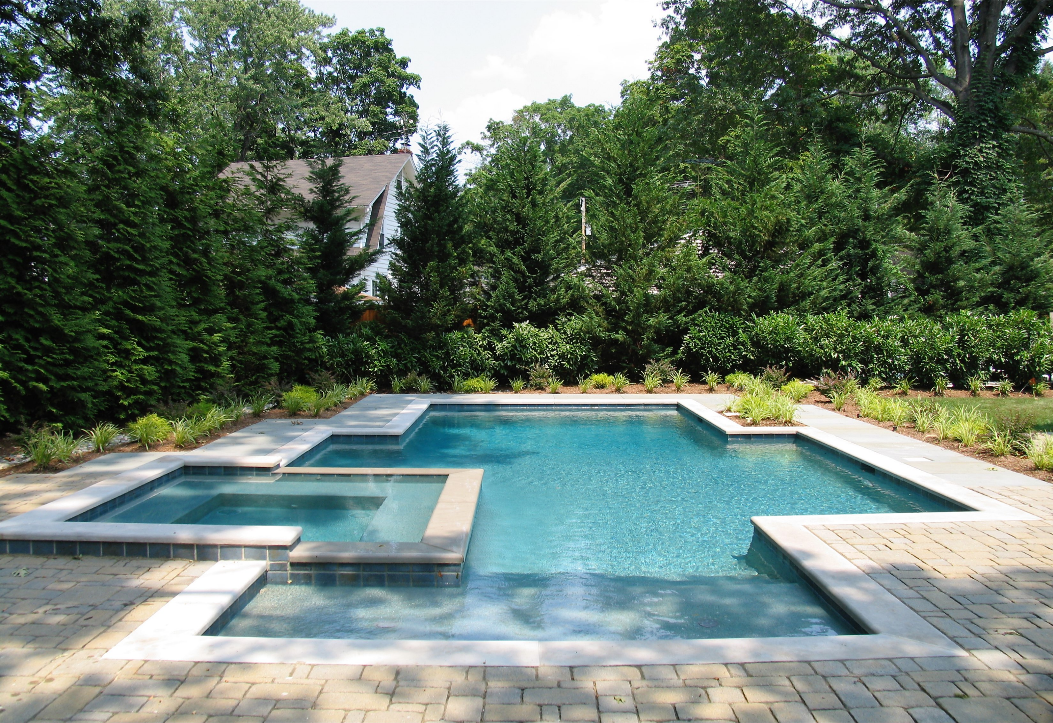
600 square foot pool/spa combination with Indiana Limestone coping, custom mosaic tile and a SeaFoam Green PebbleSheen finish.
