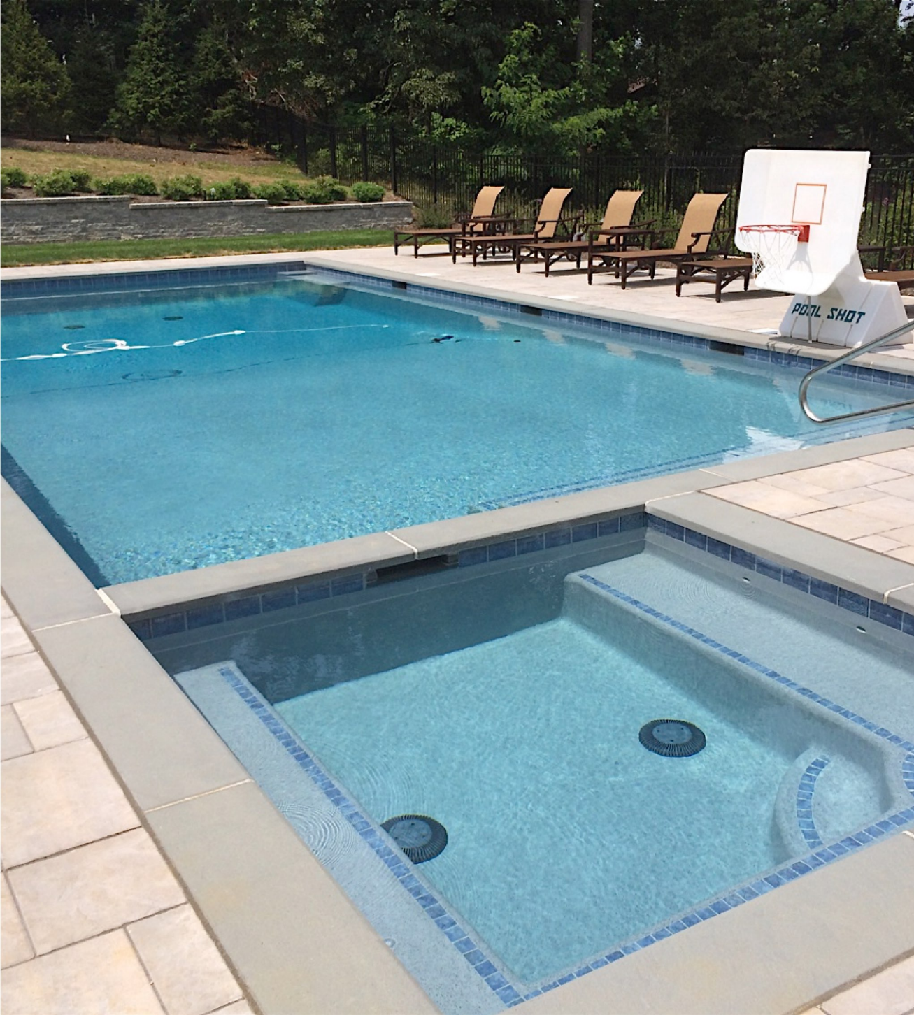
900 square foot pool/spa combo with full bullnose bluestone coping, porcelain tile, and a Hydrazzo French Grey finish.
