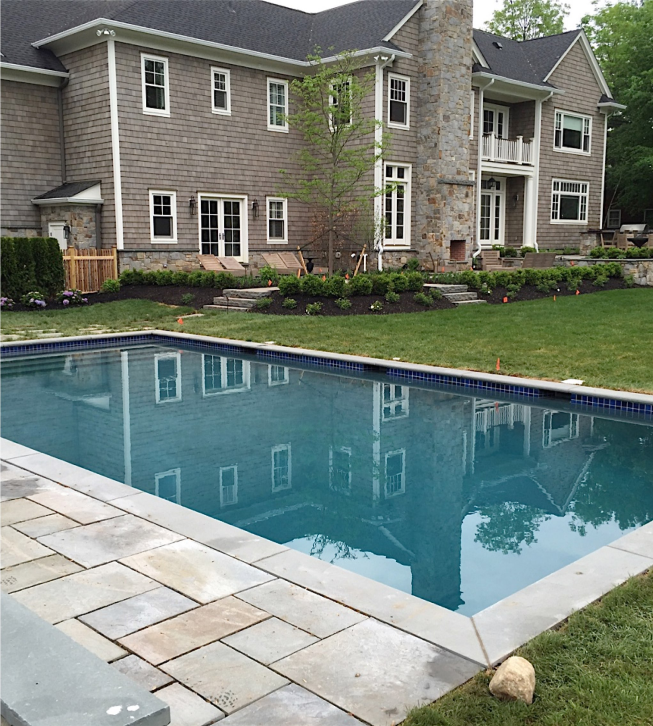
650 square foot pool with full bullnose Bluestone coping, porcelain tile and a Hydrazzo French Grey finish.
