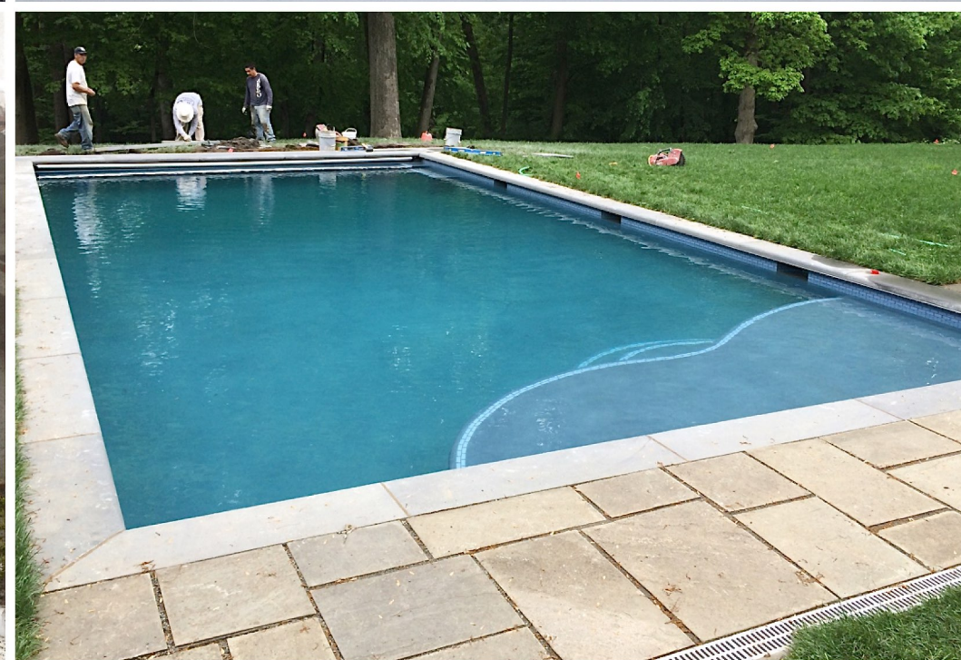
800 square foot pool with bluestone coping featuring custom glass tile, Hydrazzo Mediterranean Blue finish and a Cover Pools automatic safety cover.
