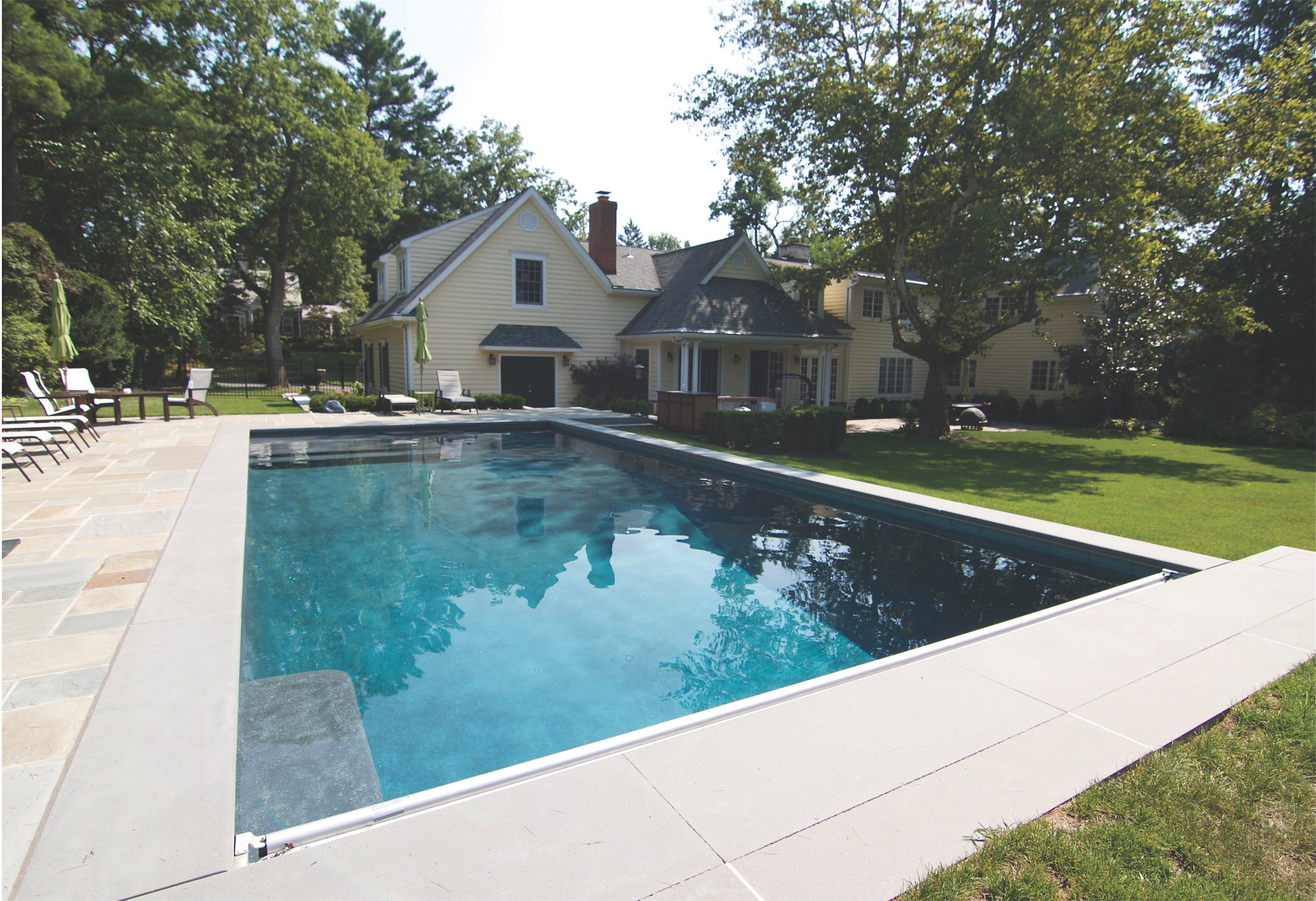
800 square foot pool with bluestone coping, custom glass tile and Hydrazzo Classico Laguna finish.
