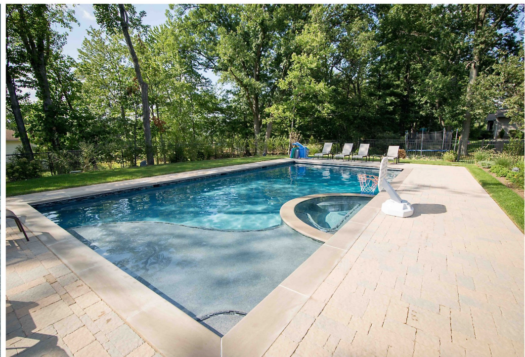
800 square foot pool/spa combination with custom glass tile, bluestone coping, a Hydrazzo Classico Patino pool finish and a Cover Pools automatic cover.
