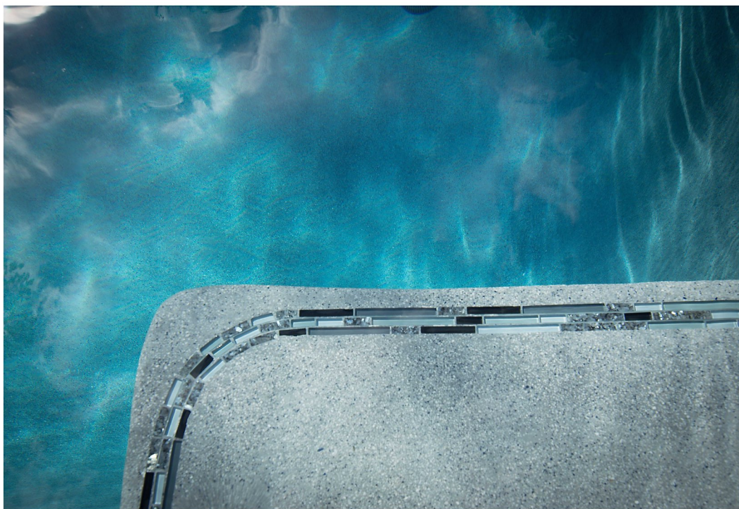
800 square foot pool/spa combination with custom glass tile, bluestone coping, a Hydrazzo Classico Patino pool finish and a Cover Pools automatic cover.
