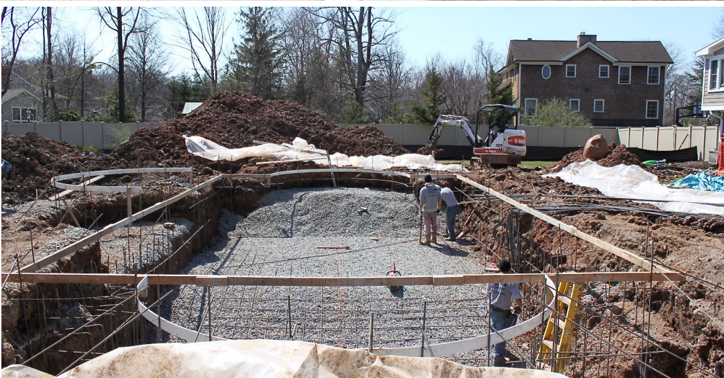
Remove old liner pool and replace with custom-designed 850 square foot gunite masterpiece. From demolition to swimming, this project took approximately ten weeks.
