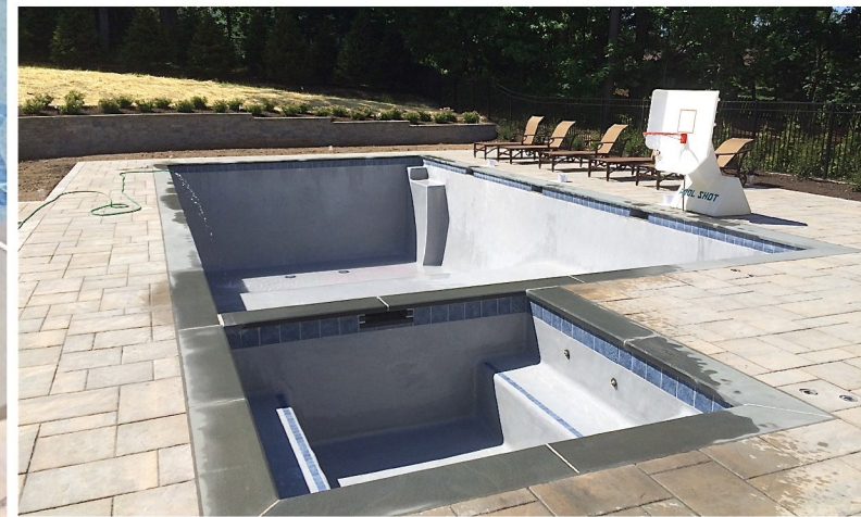
900 square foot pool/spa combo with full bullnose bluestone coping, porcelain tile, and a Hydrazzo French Grey finish.
